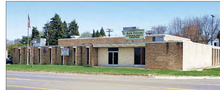
1966 brought Local 653 another brand new Union Hall at 990 Joslyn Road. These were the "Wide Track" years, with over 20,000 employees at Pontiac. The facility is still in use today as the Ruth Peterson Community Center.
